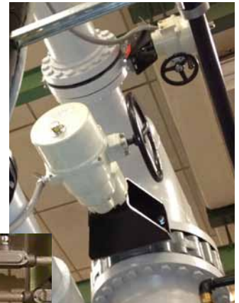
P7 Controlling Chiller Flow
